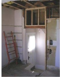
We removed a soffet that hid the original ceiling vent (above the refrigerator) someone covered it up with suspended ceiling tiles. By the time the wall was removed, the whole ceiling came down.
