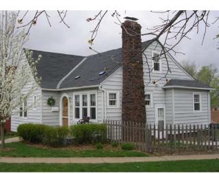
Peter and I replaced all the storms and I re-glazed most the windows . We replaced the basement doorsill and the storm door. That first spring, I noticed in the basement walls were damp. We added a gutter above the dormer, and replaced the front gutter. We re-graded around the perimeter of the house and solved the damp wall problem in the basement.
